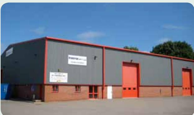
Transvac's new Research & Development Facility
